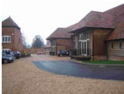
A recent conversion of agricultural buildings into business premises
